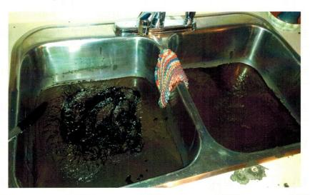
This is a severe affected area from **Grease** being thrown down the drain.
